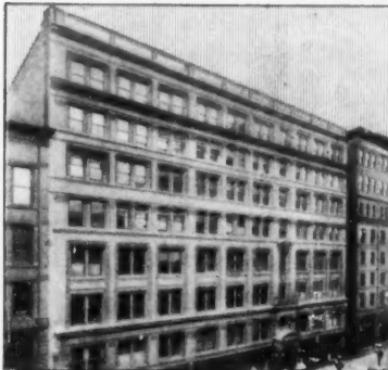
Barrett Specification 20-Year Bonded Roof on Connell Estate, Scranton, Pa. Roofer: Globe Slag Roofing Company, Scranton, Pa.
